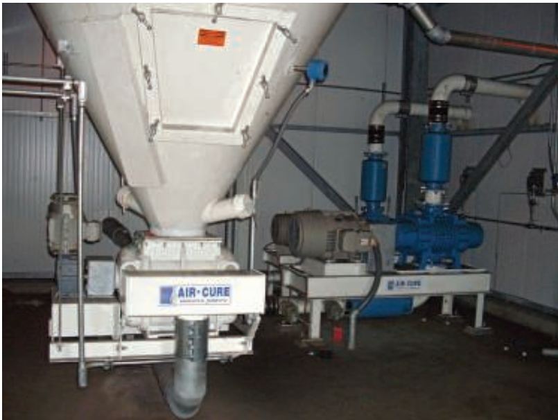
5. Dustless option. A dust hopper with a pneumatic conveying system. Courtesy: Air-Cure Inc.
