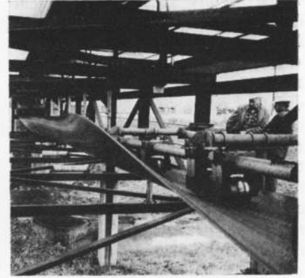
Fig. 11 — Belt turnover at American Electric Power Co.'s James M. Gavin power plant, Cheshire, Ohio.
