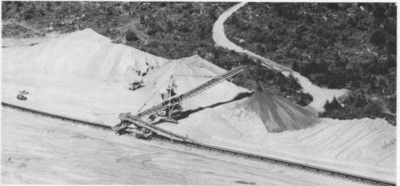
View of tripper and spreading stacker at Washington Irrigation & Development's coal operation, Centralia, Wash.
