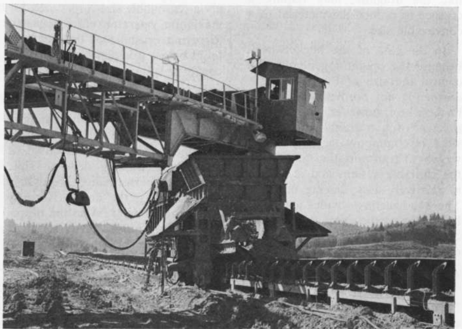
Fig. 1 — Traveling impact section used at Washington Irrigation & Development's coal operation at Centralia, Wash.
